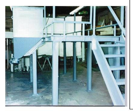
This picture shows a working platform serving aggregate bins. Notice the comfortable steps leading to the solid steel deck and the removable railing built to OSHA specifications. The platform was fabricated in modular form ready to be assembled at the job site with simple tools.
